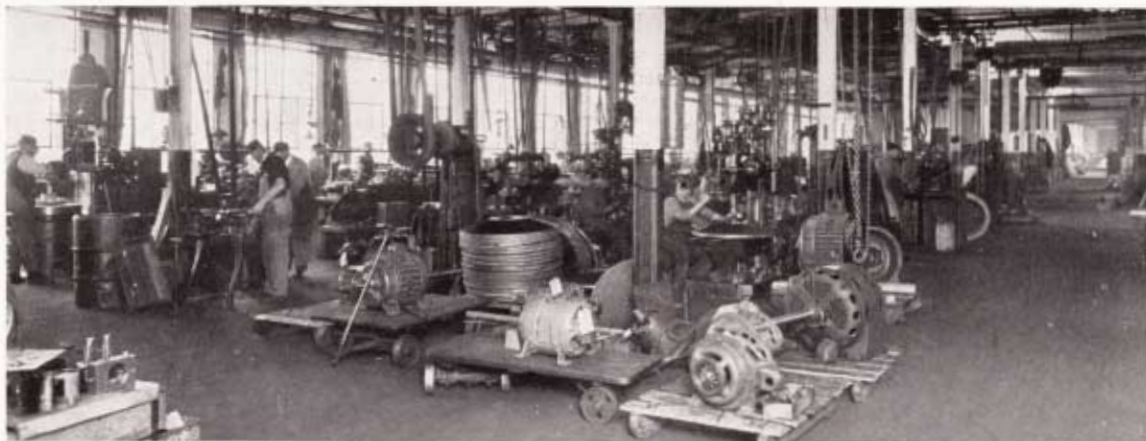
One corner of the Spencer Machine Room
